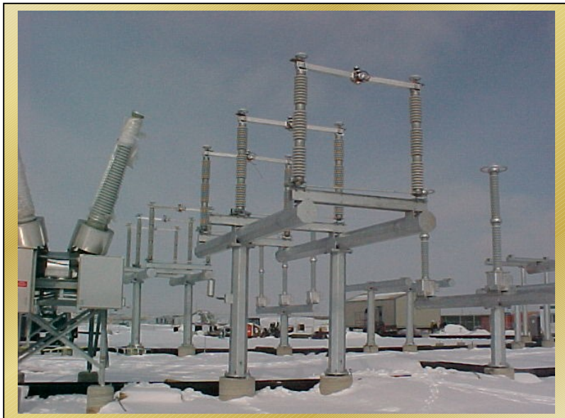
EC-1 245 kV, 3000 Amperes Switch Installation In Progress
