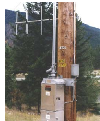
145 kV LLS-II-2000 Mounted On Steel Unitizing Frame And Driven By A VM-1SE.
