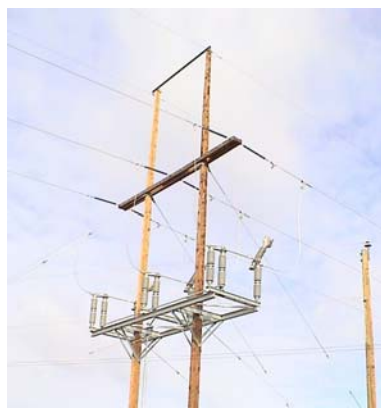
145 kV LLS-II-2000 Mounted On Steel Unitizing Frame And Driven By A VM-1SE.
