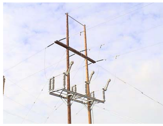
145 kV LLS-II-2000 Mounted On Steel Unitizing Frame And Driven By A VM-1SE.
